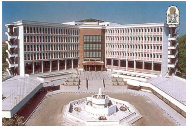
Administrative building of Assiut University
