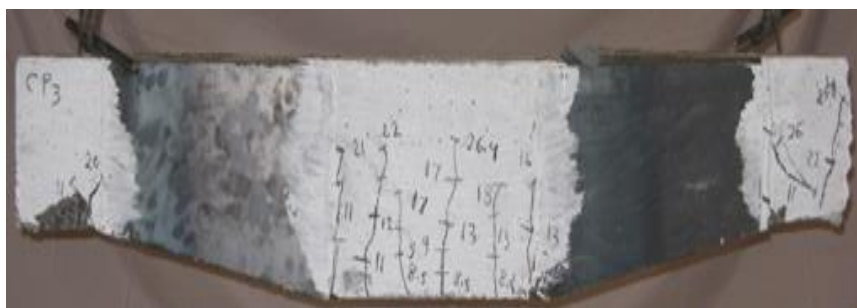
Fig. (35): Crack pattern of beam "CP.3" with thickness of steel plate (2.00 mm)
