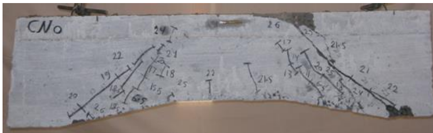
Fig. (2):Crack pattern of beam "CN.0".
