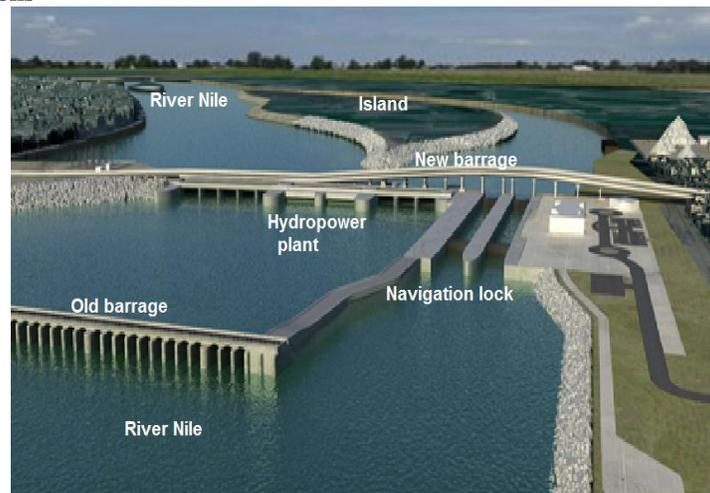
*Figure (1):* The proposed project of New Assiut Barrage and its Hydropower plant
